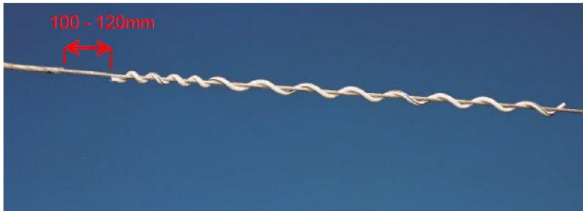
Figure 6 – SVD Installation Location
